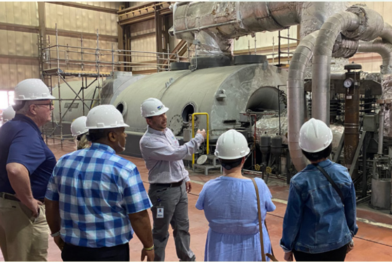
Members of the KS legislature and Congressional staff tour Nearman Power Plant learning how policy decisions affect public utility services.
